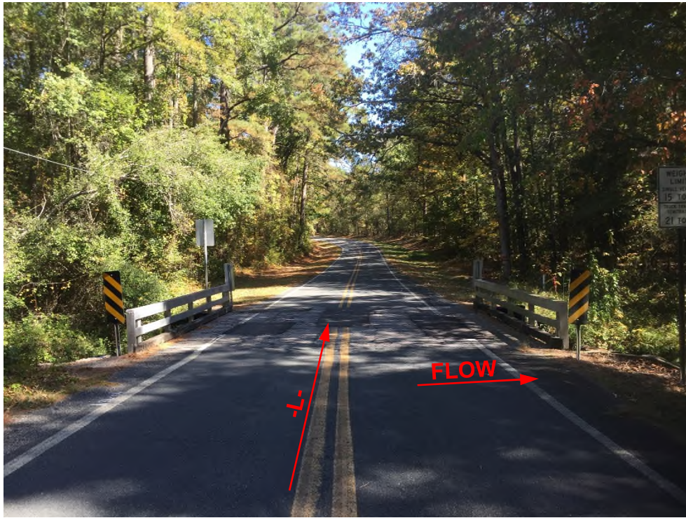
Photograph No. 2: View of -L- and Rocky Fork Creek looking east.
